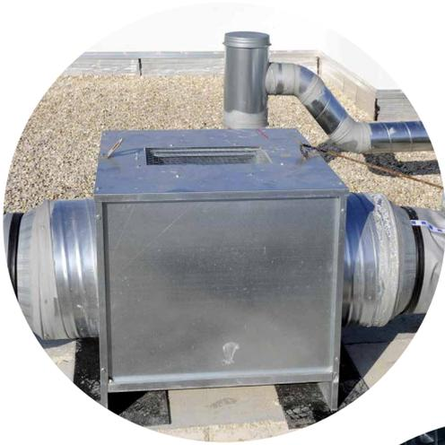
When positioned on a ventilation box, the Delta P lets one monitor, at a distance, the proper operation of the system, and it will be alerted in the event of a malfunction (electrical, breakdown, fouling...).
